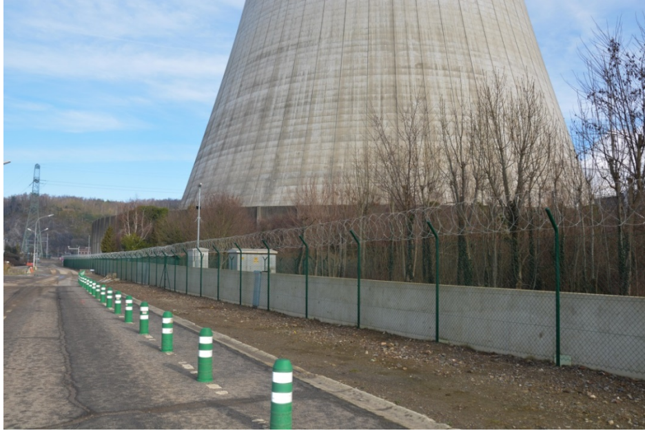
Figure 3: Peripheral protection of the site of Tihange against beyond-design flooding realized in 2015
