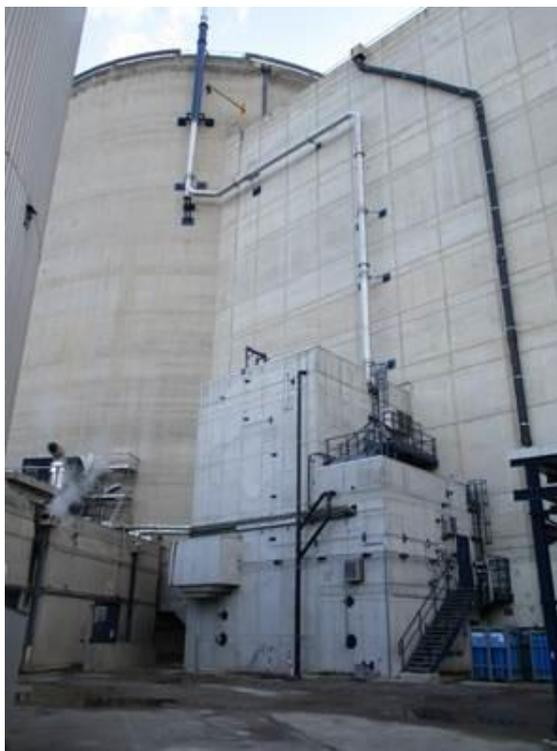
Figure 7 : Filtered containment venting systems of Tihange 3
