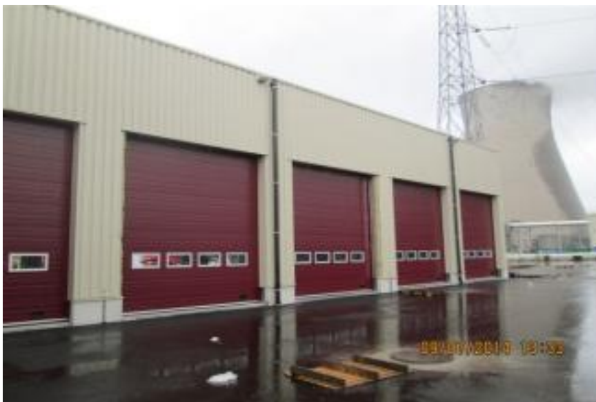
Figure 9 : Construction completed of the new storage building at Doel NPP.
