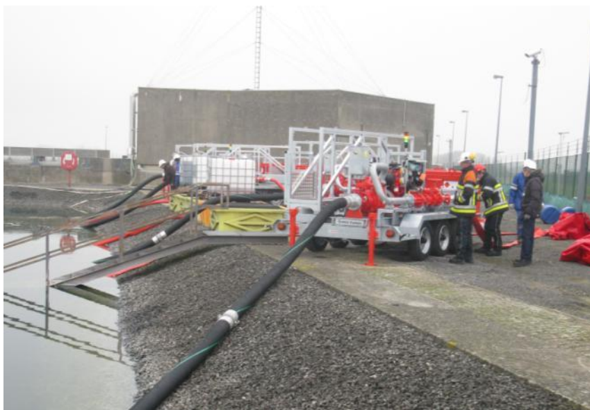
Figure 6 : Mobile pumps training at the Doel NPP in the framework of the CSBO strategy
