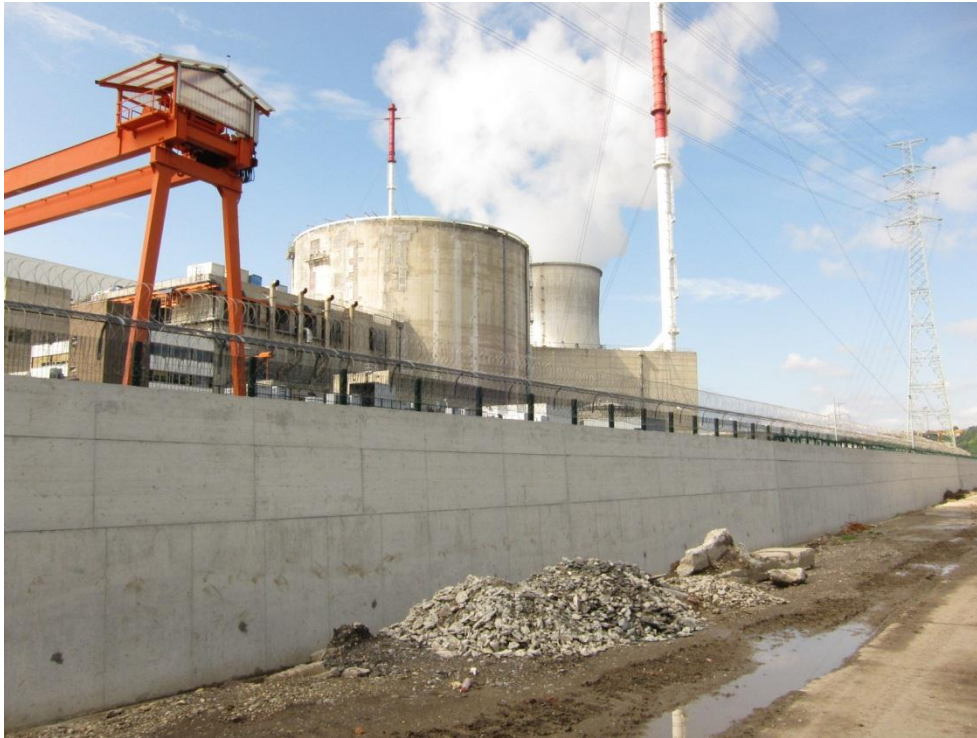
Figure 2: Peripheral protection of the site of Tihange against beyond-design flooding
