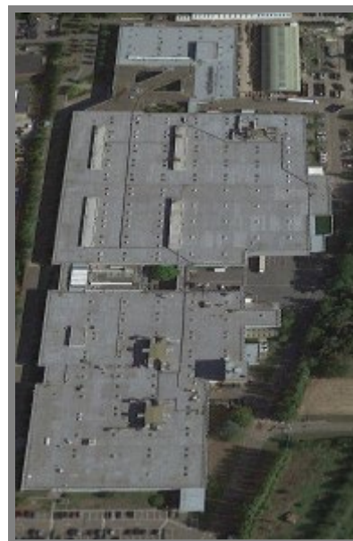
Figure 2 CommScope à Kessel-Lo
