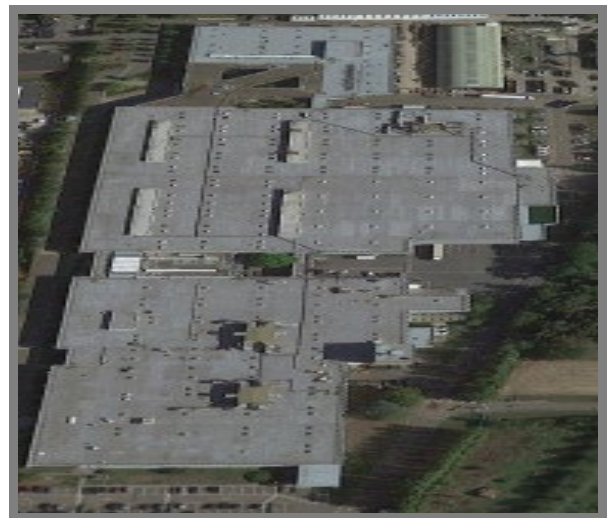
Figure 1 CommScope à Kessel-Lo
