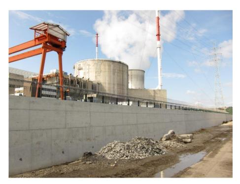
Figure 2: Peripheral protection of the site of Tihange against beyond-design flooding realized in 2015
